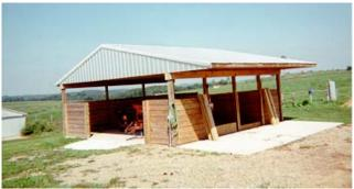
Figure 3. Four Bin Arrangement for Poultry Mortality. Bins are for primary (2), secondary and amendment storage. Additional space is for storage of material prior to land application.
